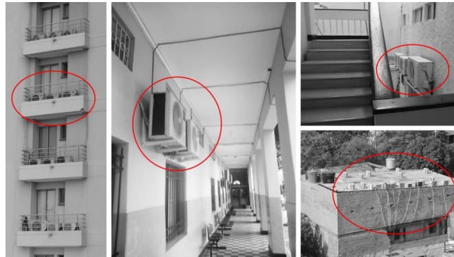
Figure 2. Example of balconies and other spaces used to house air conditioning equipment.
